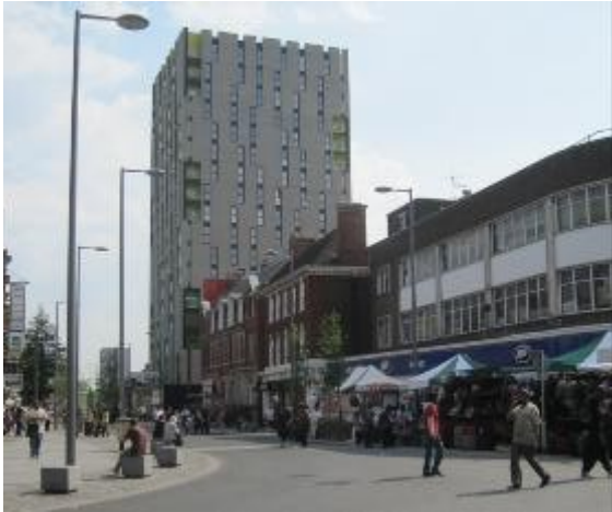
New paving, street furniture and a new road layout to accommodate the new ELT1 at the southern end of Station Parade and Ripple Road.
