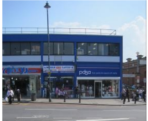
Poor quality building stock does not have a positive impact on the character of Station Parade.
