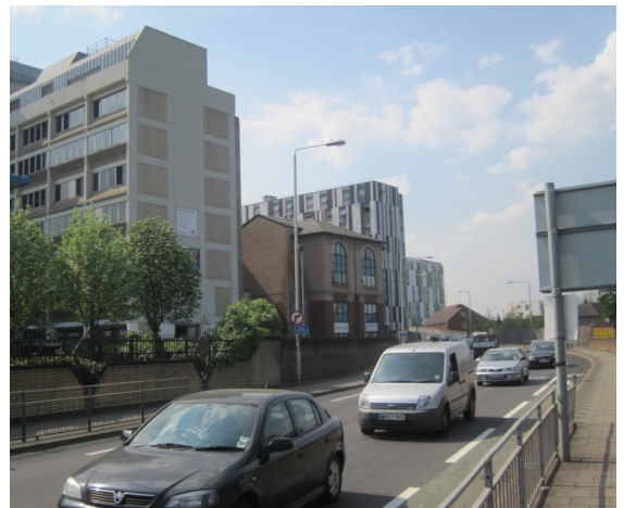
Barking edges. The north-west corner of the Masterplan area is poorly defined.
