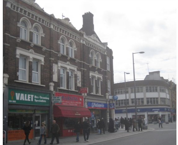
The fine street grain of Station Parade needs to be maintained and enhanced to ensure connectivity and local character is retained.
