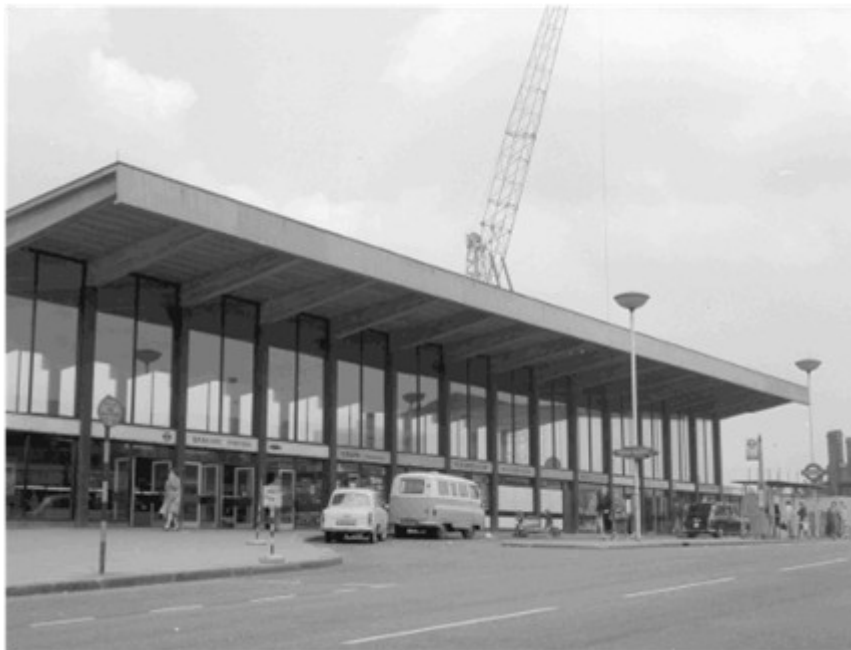
Figure 8: Barking Station shortly after completion in 1961
